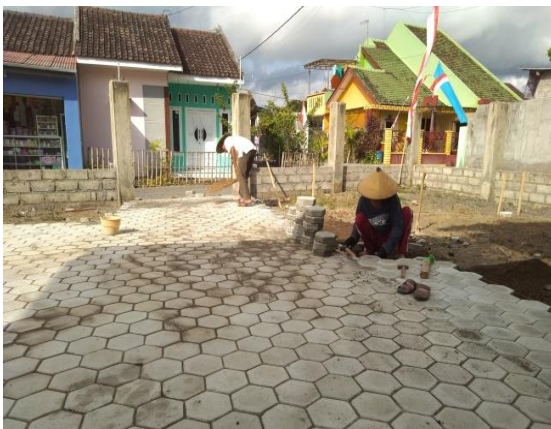
Gambar 10 Proses pemasangan paving halaman mushollah
