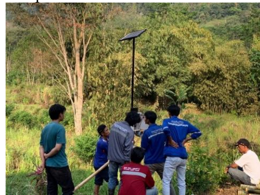
Gambar 6. Proses Pemasangan Alat Early Warning System dan Panel Surya
