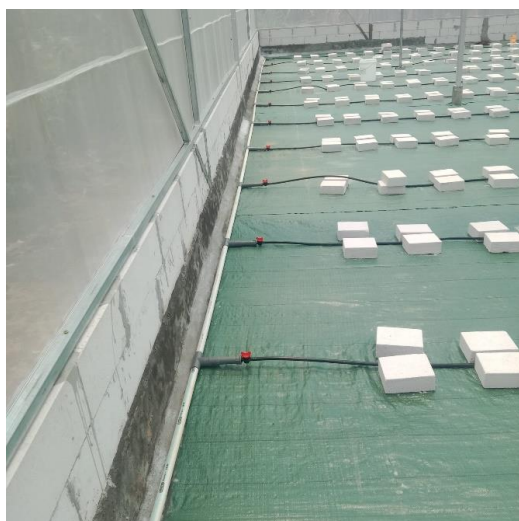
Gambar 1. Proses persiapan perpipaan
