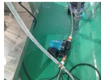
Gambar 3. Pompa Booster
